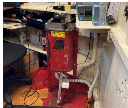
Carousel controller (ex MTT tram controller).
