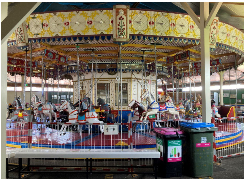
Overall view of carousel, showing centre console, pressed metal rounding boards (top), platform and horses.
