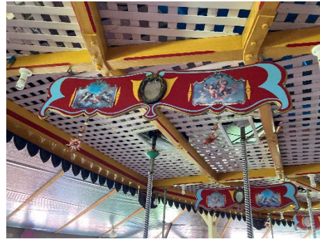
Sweeps, quarterings, lattice ceiling [original fabric] with drop panels [not original fabric].
