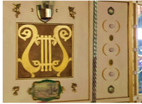
Original speaker aperture with decorative fretwork inserts (lyre motif) and cloth backing.
