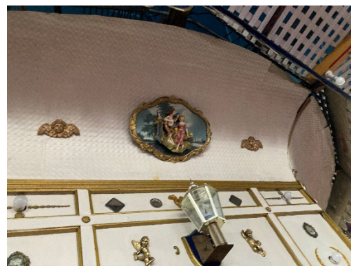
Pressed metal soffit to centre console, with applied decoration [not original fabric].
