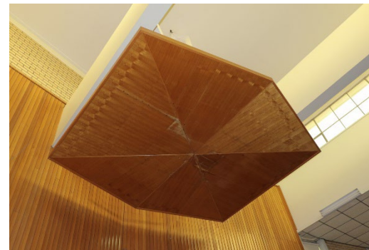
Underside of baldachin showing water damage
