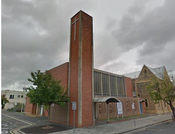
Former North Adelaide Memorial Methodist Church, North Adelaide, 1963
