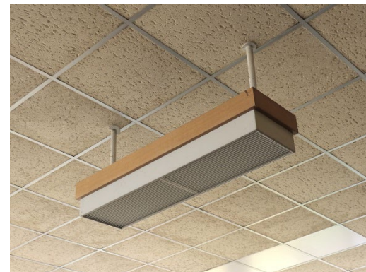
Flourescent light enclosure and suspended ceiling
