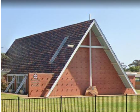
Former Salisbury Methodist Church, 1961, is an example of a true A-frame church
