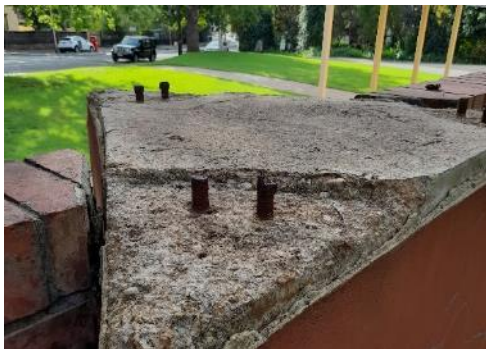
Reinforced concrete base of toppled spire
