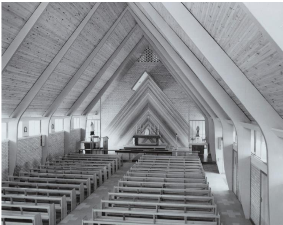
St John Vianney's Catholic Church, interior c.1962, showing portal frames and matchboard ceiling, note the triangular detailing to reredos.
