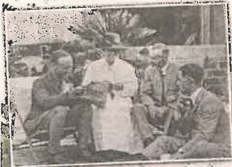
Dilapidated historic mansion Aviemore, former family home of Sir Ross and Sir Keith Smith, inset on the verandah with their parents, faces the wrecking ball. Pictures: Dean Martin, State Library of SA
