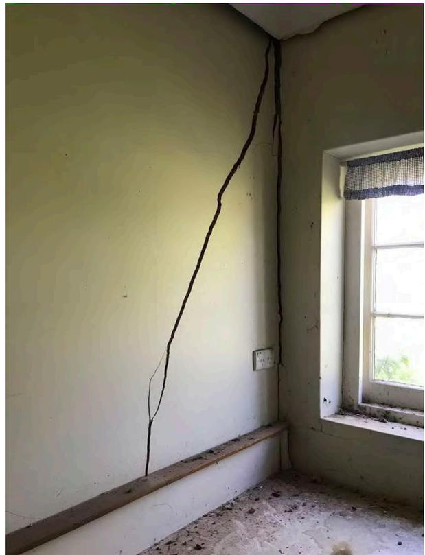
Figure 17: Cracking to masonry walls and interior of (former) kitchen wing
