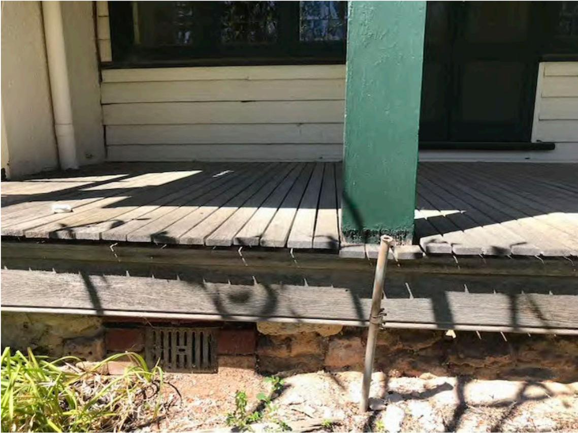
Figure 24: Subfloor masonry walling to verandah of single-storey wing
