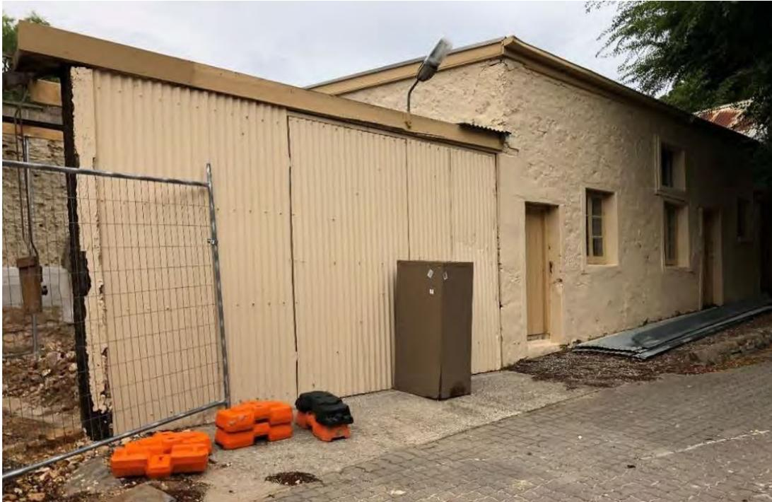
Figure 13: outbuilding with lightweight addition to older masonry section; collapsed wall at left (GGA, February 2021)
