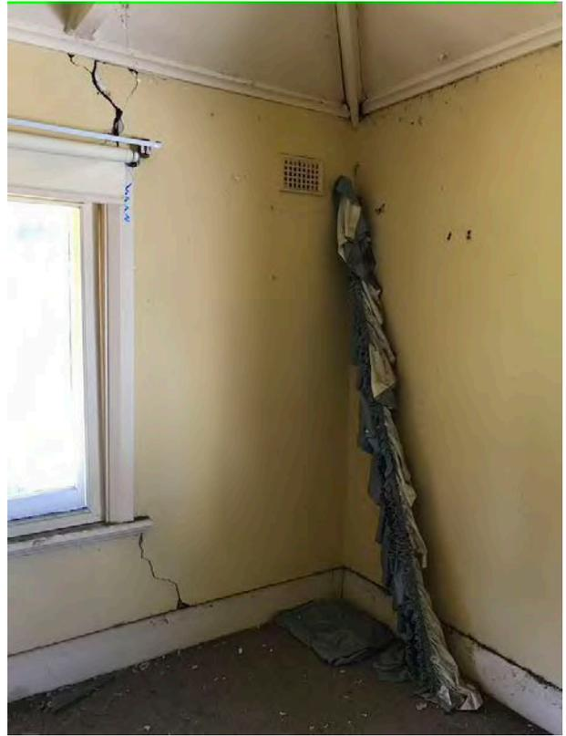
Figure 22: Damage to masonry walls of double-storey wing
