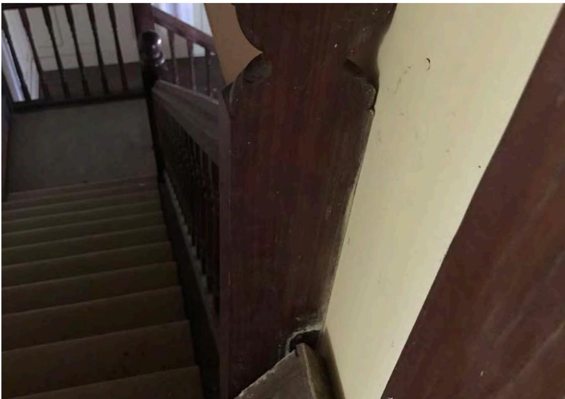
Figure 16: Incongruous fitting of internal stair with half newel post
