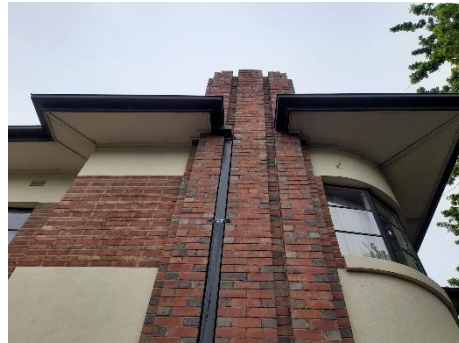
Tower containing chimney
