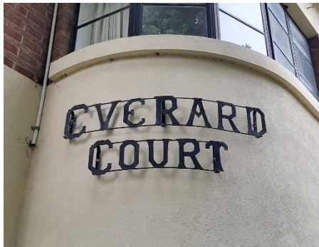
Steel plate and rod lettering
