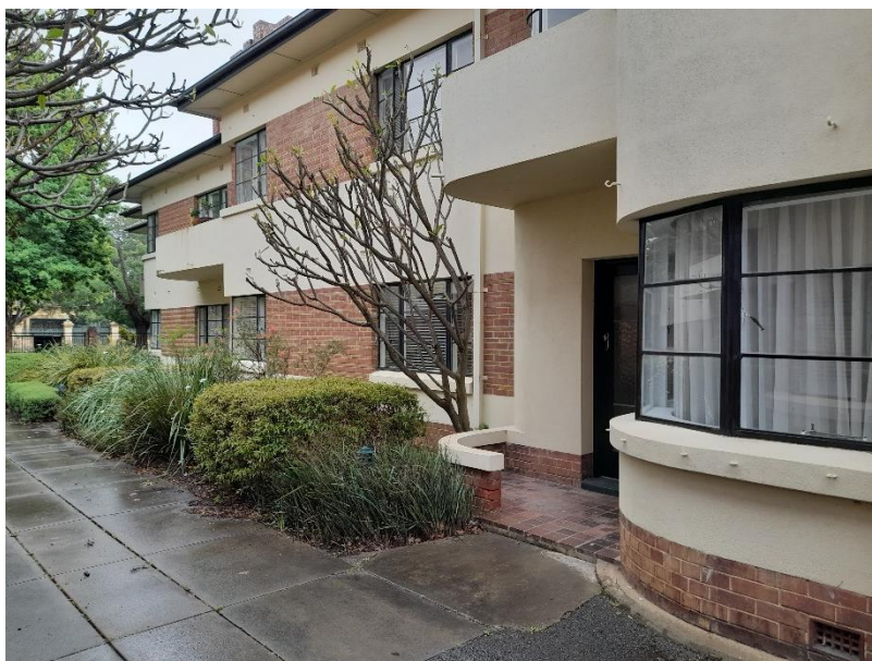
East Wing, view towards Anzac Highway
