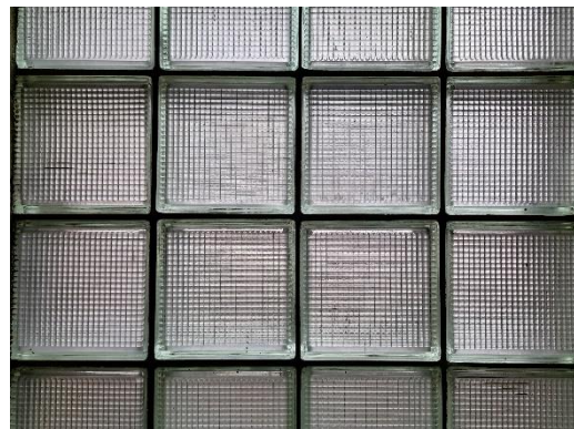
Glass bricks to internal stairwell
