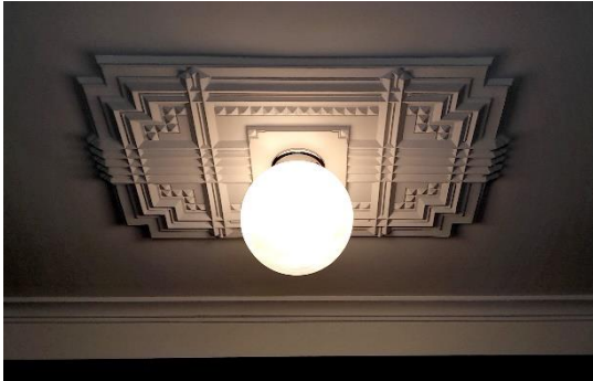
Typical ceiling rose
