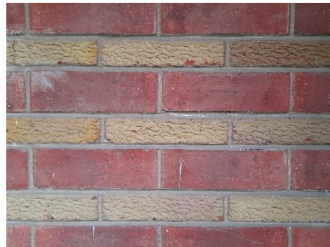
Standard red and yellow Roman vermiculated brick coursing
