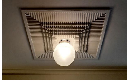
Typical ceiling rose
