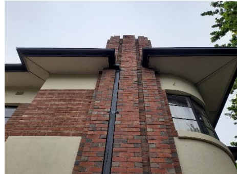
Tower containing chimney
