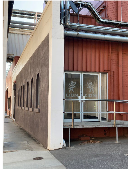
Walkerville Brewhouse Tower showing the addition to the front for the museum exhibition space.
