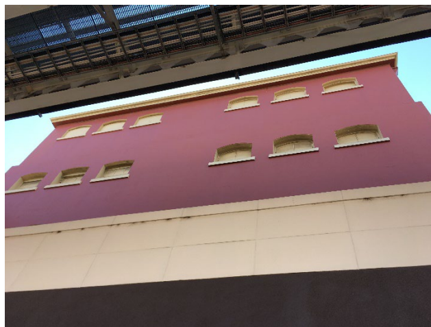
Southern elevation (facing Winwood Street now closed)
