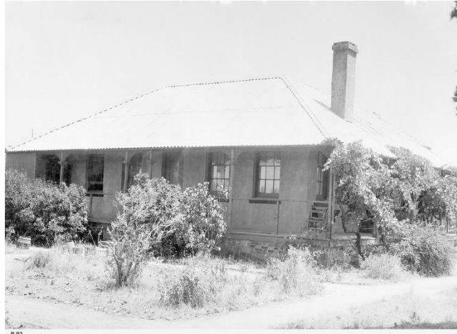
Front of Theberton Cottage c.1923, Tregenza suggests this portion of the building formed 2 of the 4 rooms of the original structure, however, it lacks the 'lofty' dimensions of the building behind and may have been a later addition.
