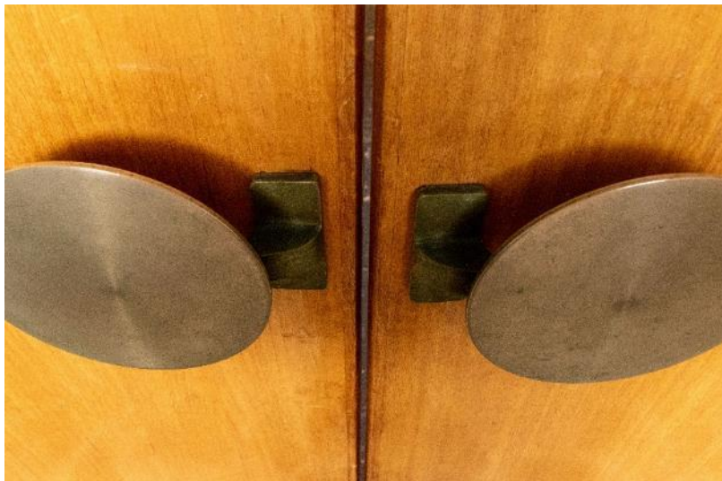
Narthex door handles in cast aluminium Source: DEW Files 28 January 2021
