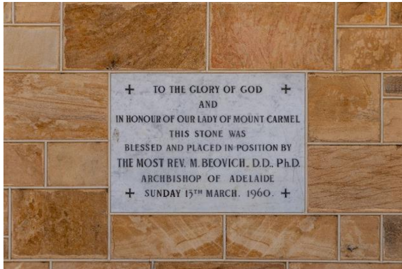
Foundation stone showing sawn basket range stone facade
