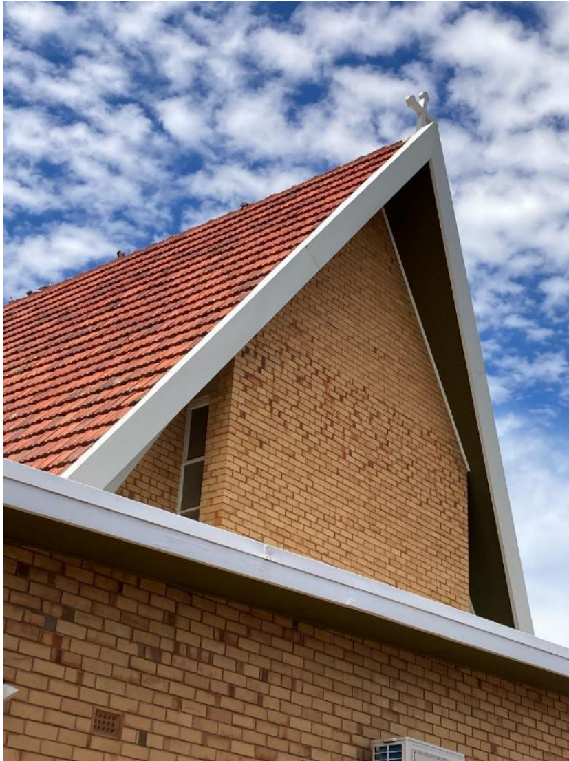
Rear (north) gable
