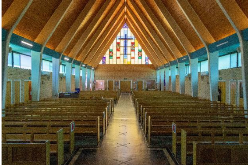
Interior nave looking south Source: DEW Files 28 January 2021
