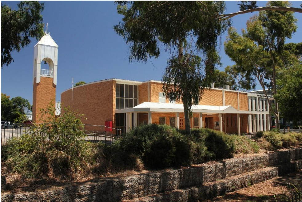
View from northeast showing tower; note post-1999 tower belfry
