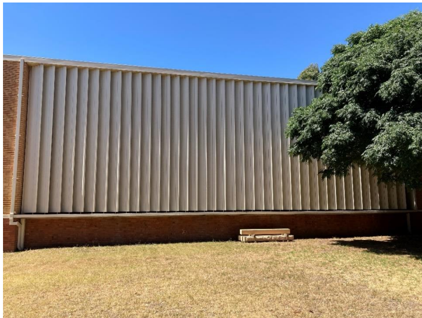
South-western side showing fixed louvres
