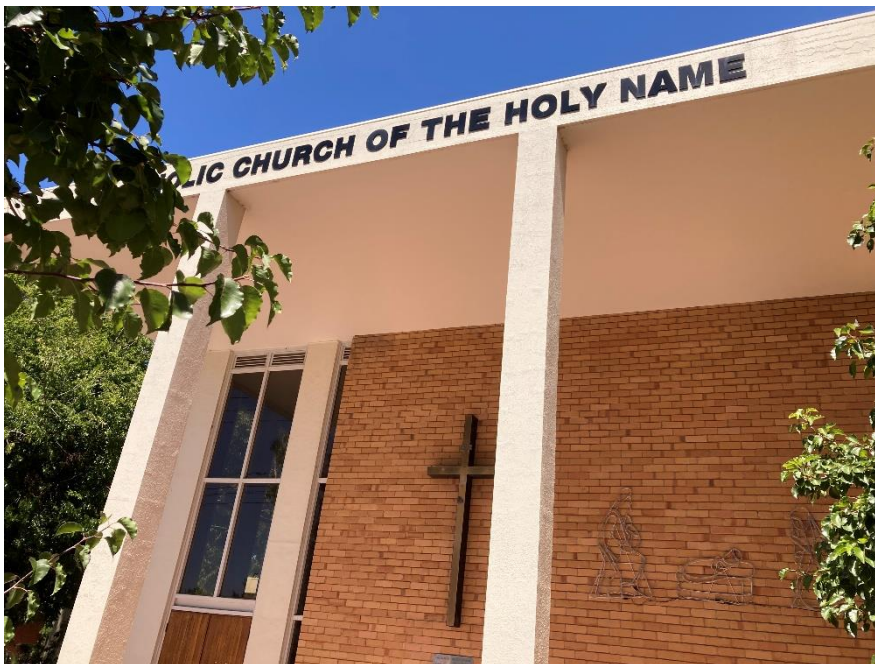
Colonnade detail facing Payneham Road with contemporary laser-cut lettering
