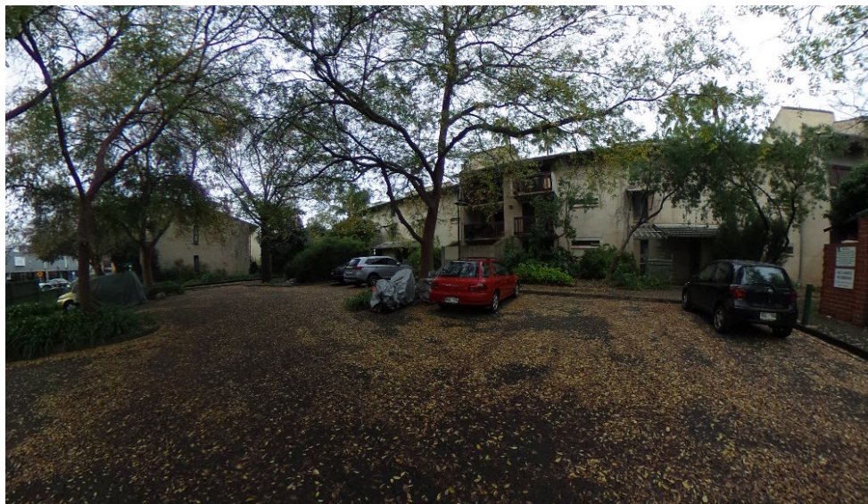
Dr Kent's Paddock 3-storey flats, viewed from car park fronting Rundle Street, looking east to cottage flats for pensioners.
