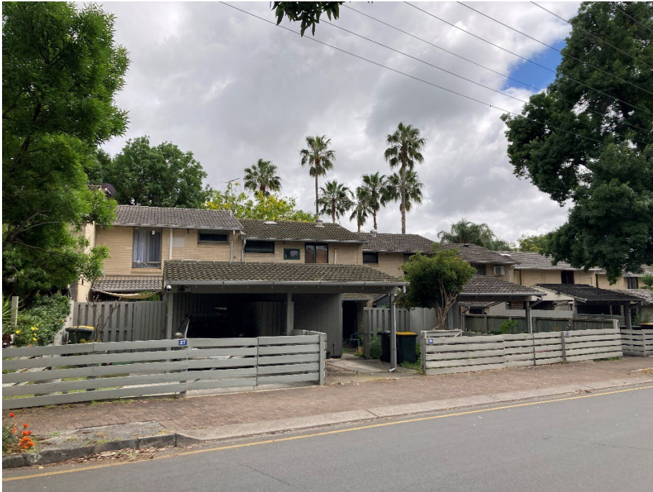
Townhouses to Capper Street, note the stepped siting to accommodate the block shape.
