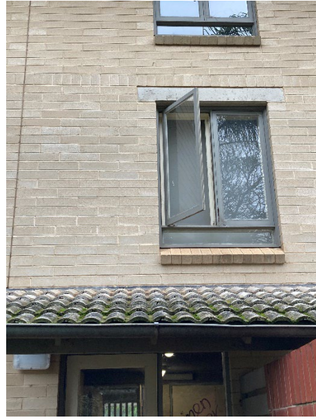
Flats showing window details, note concrete lintel, band of brick above, brick sill and concrete tiles to roof.
