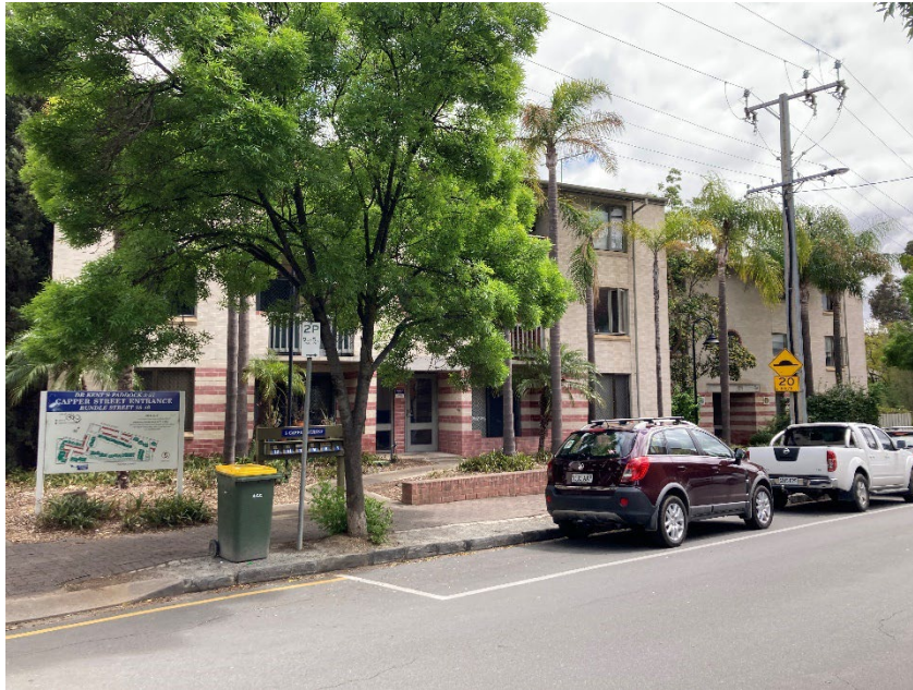
Stage 2 flats fronting Capper Street.
