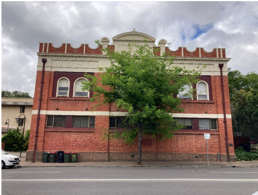
Former John Martin's Warehouse.
