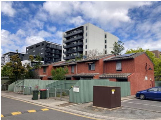
Box Factory, Carrington & Regent Streets, Adelaide showing 2-storey flats (top left), 3-storey flats (top right) and townhouses (bottom left).
