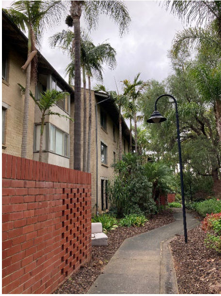
3-storey flats fronting communal garden, note the red brick wall.
