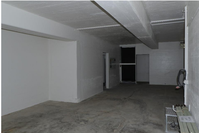
General interior view DEW Files 4 February 2021
