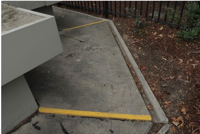
Original cement paving and integrated drain
