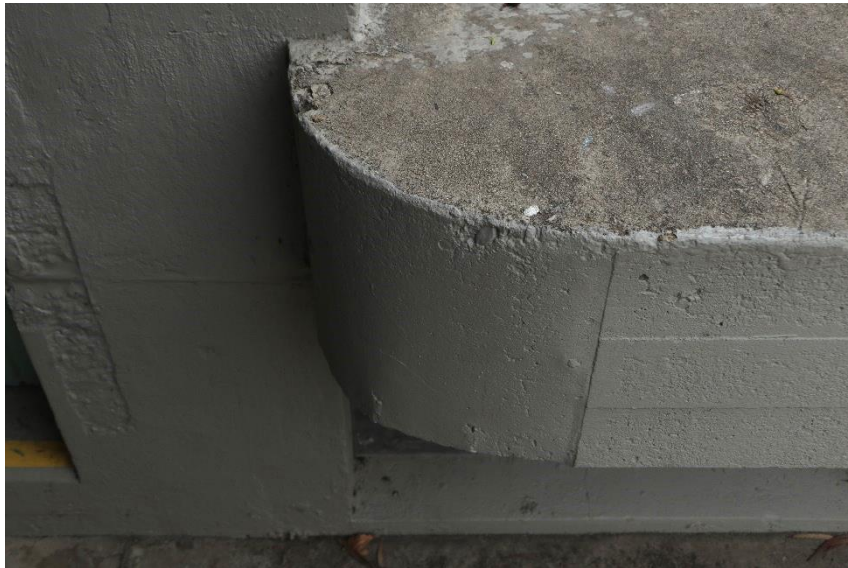
Detail of board-formed concrete
