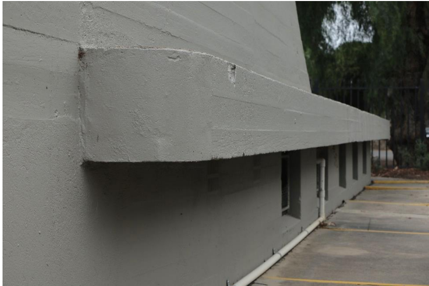
Side view showing windows
