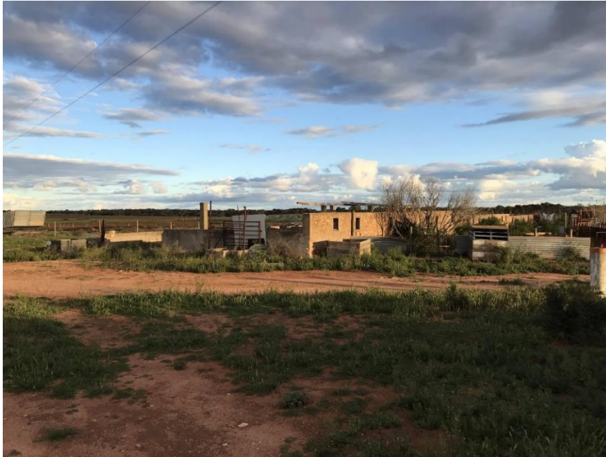
Northern elevation of the piggery breeding pens
