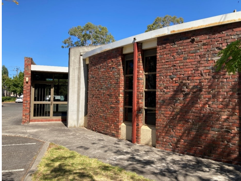
North-eastern side of church showing rear porch, portal frame and clinker brick walls
