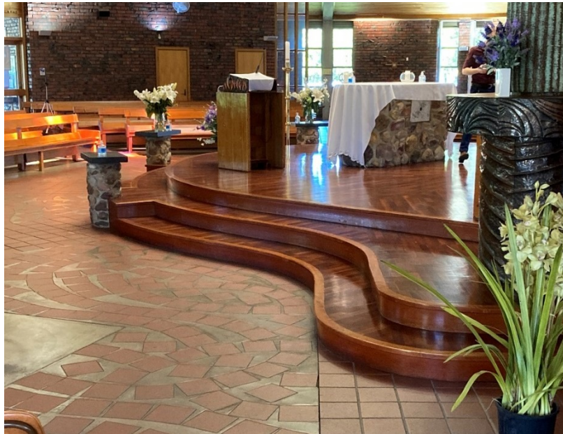
Floor of nave and sanctuary showing quarry tiles and timber mouldings
