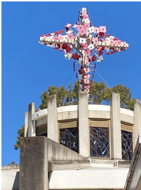
Roof lantern and 'Great Cross' Source: DEW Files 21 January 2021
