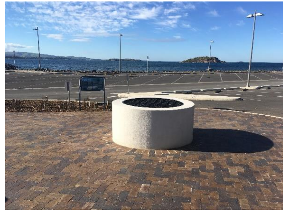
Site works complete June 2019 Source DEW
