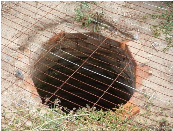
Uncovered well 23 November 2017 Source DEW
