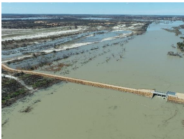
Pike regulator in operation during 2022.
