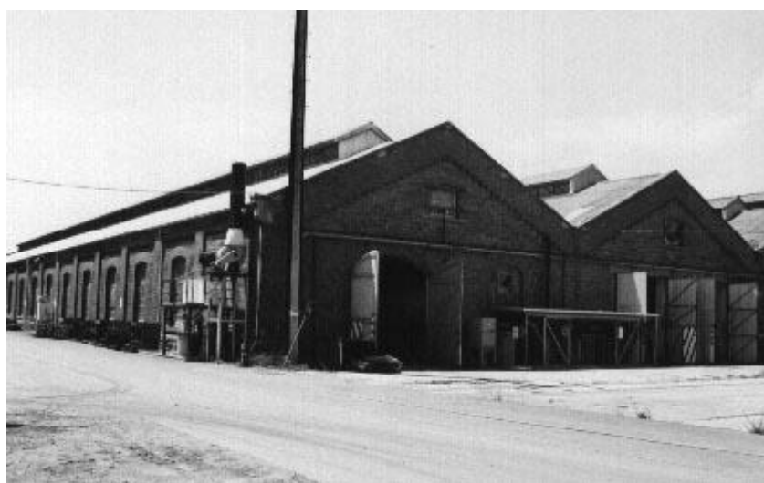
Figure 2. Fabrication Shop SHP 14686
