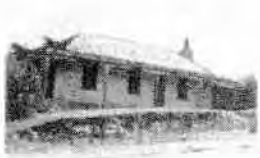
Cottage 31 has original flat iron roofing
