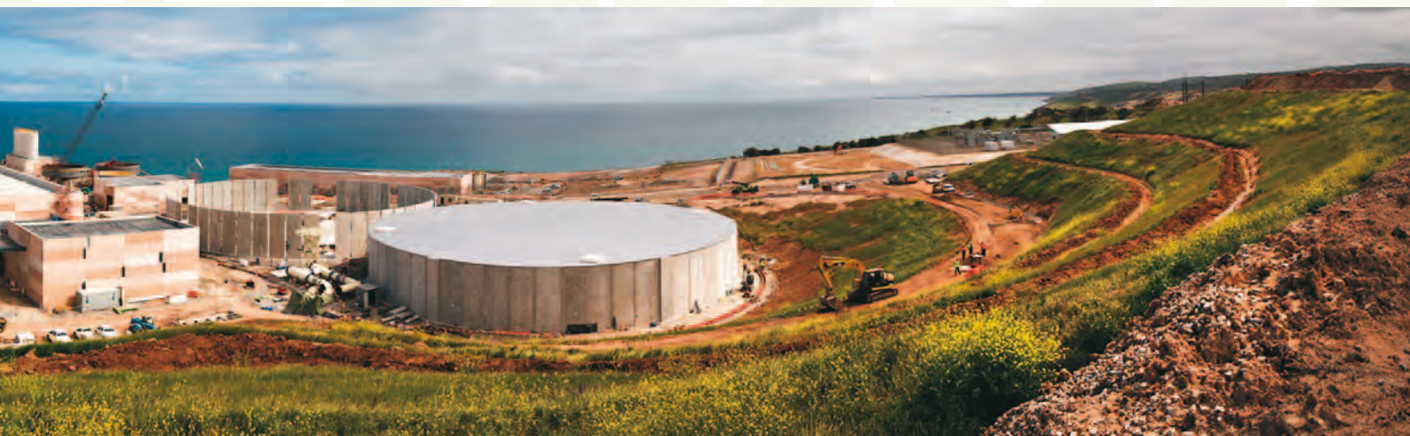
The Adelaide Desalination Plant, being constructed at Port Stanvac, is due to start producing water in 2011.
