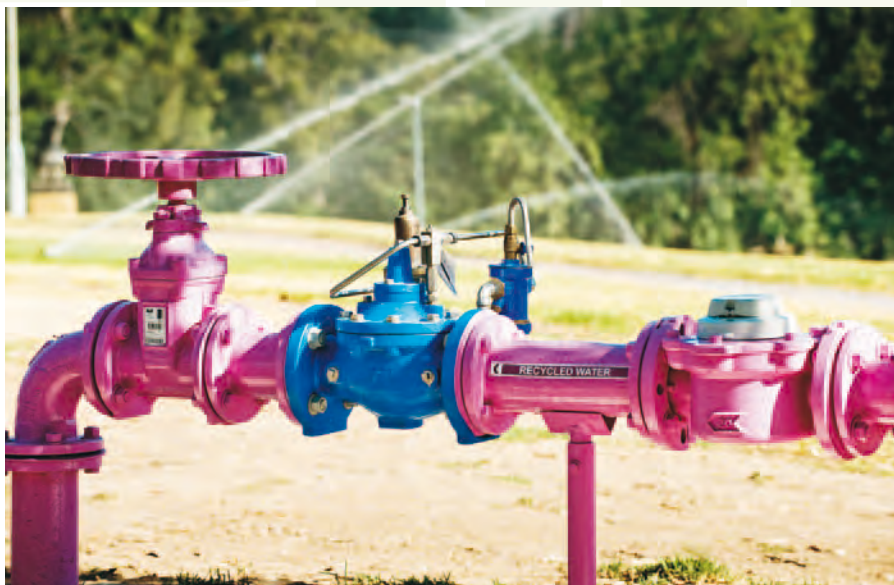
A 32-kilometre network of recycled water pipes is providing recycled water from the Glenelg Wastewater Treatment Plant to the city's parks and gardens.
