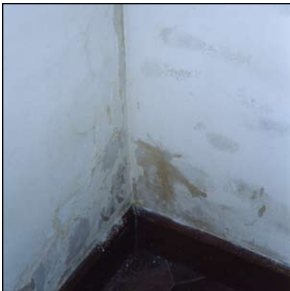
Efflorescent powdering on wall surface indicates active salt damp attack
