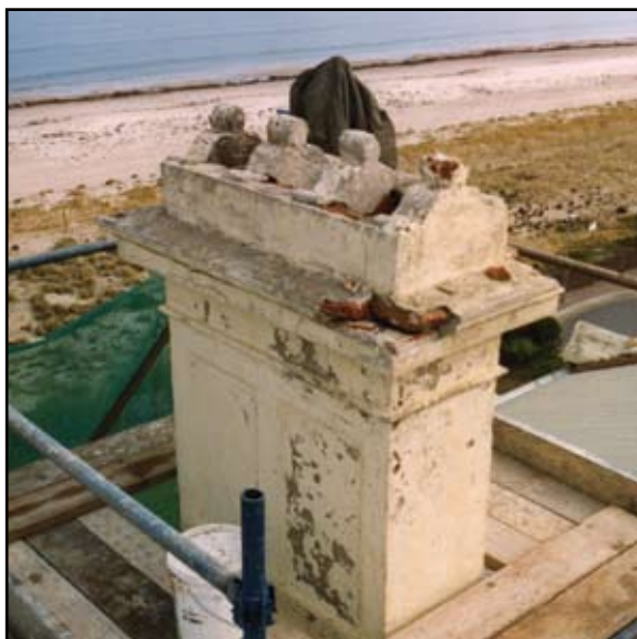
Check the condition of chimneys while on the roof. The erosion of these mortar joints will lead to eventual collapse of the brickwork. This chimney should be repointed using a traditional lime mortar mix.
