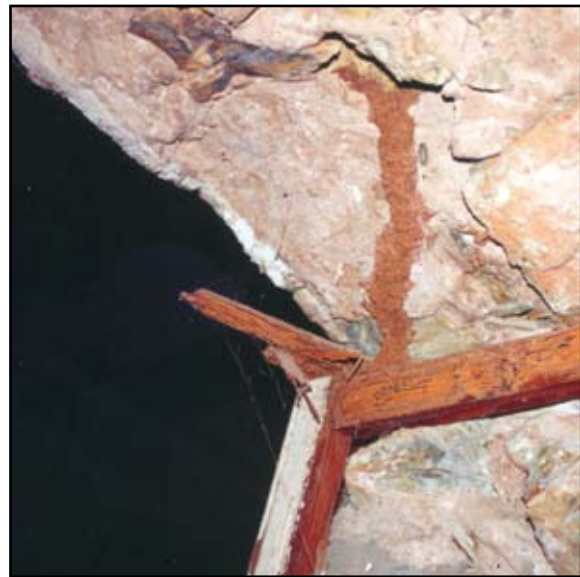
The door frame, lining and structural timber lintel of this doorway have been completely eaten by termites. A mud gallery is clearly visible at the centre of the picture.
