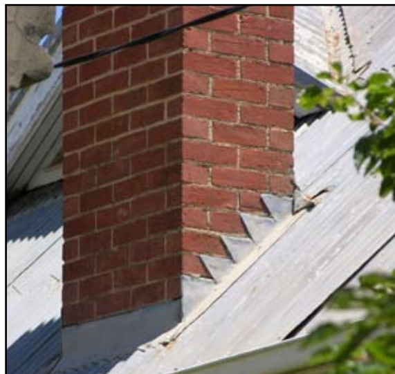
Typical chimney flashings.
