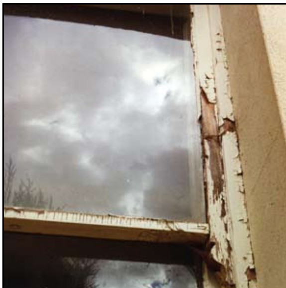
Peeling of paintwork is allowing rapid moisture damage to the window frame.
