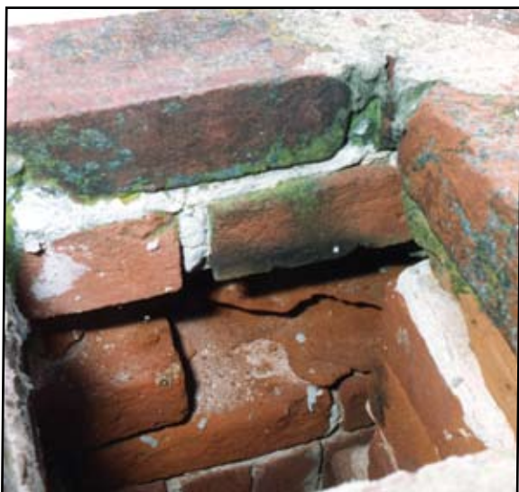
High rate of airflow up chimney has caused severe salt attack inside the flue, which is not visible from the outside.
