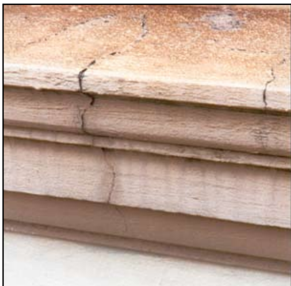
These fine cracks are sufficient to allow in water and eventually lead to the structural failure of this decorative cornice.
