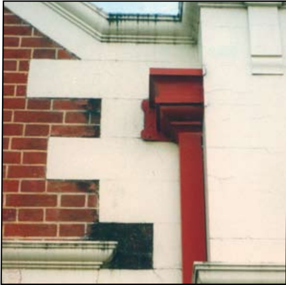
A blocked gutter and rainwater head have overflowed and saturated the surrounding brickwork, encouraging the growth of an unsightly fungal stain. Overflow such as this can also deposit harmful salts, resulting in salt attack of the masonry.
