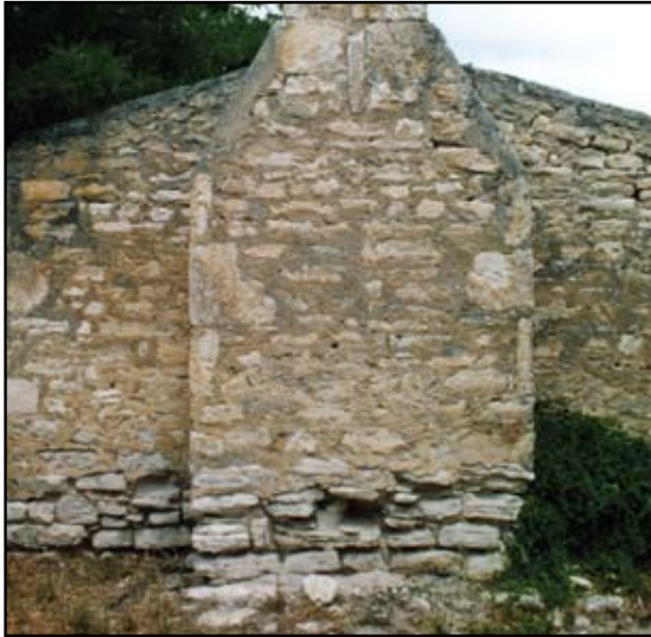
Typical case of rising damp due to lack of damp proof course.
