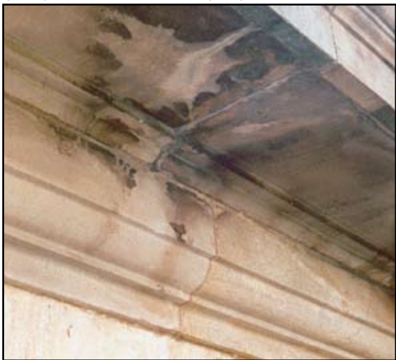
Mortar has been eroded from the joints in this stone cornice by the penetration of moisture through the top surface. Failure to repoint the joints has caused considerable damage to the stone either side of the joints. The damage is a form of salt attack due to air movement through the open joints in the presence of salts (from bird droppings for instance)
