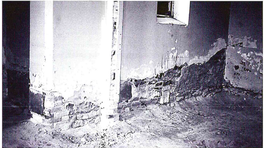
above: Rising damp on Church walls.
