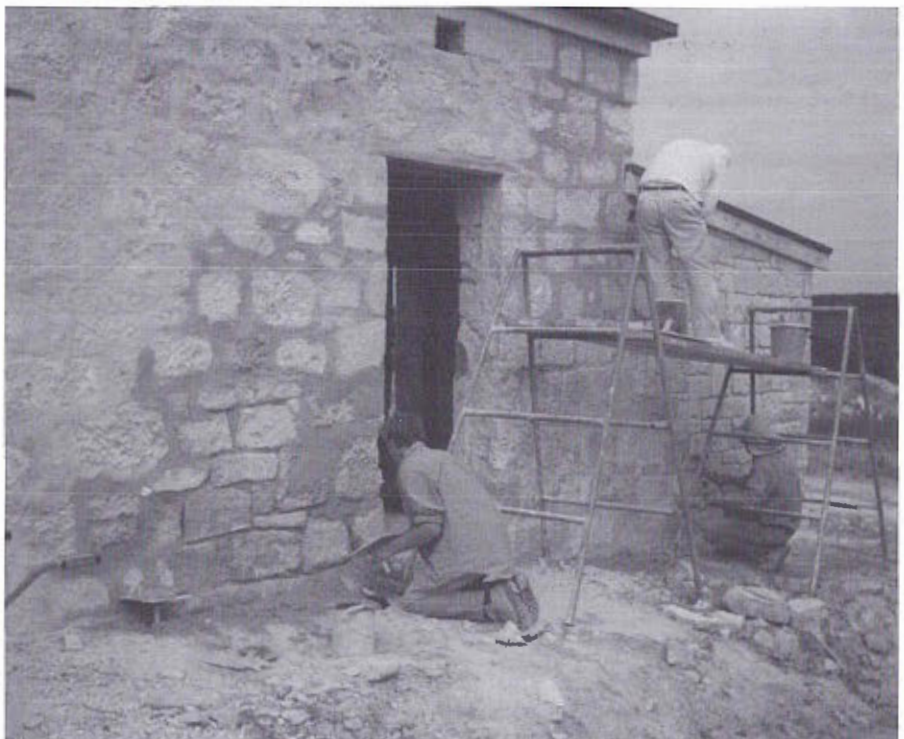
Repointing with soft mortar with the help of Green Corp. P Martinsen (top), Mathew Sparrow (bottom left), and Adam Krahnert.
