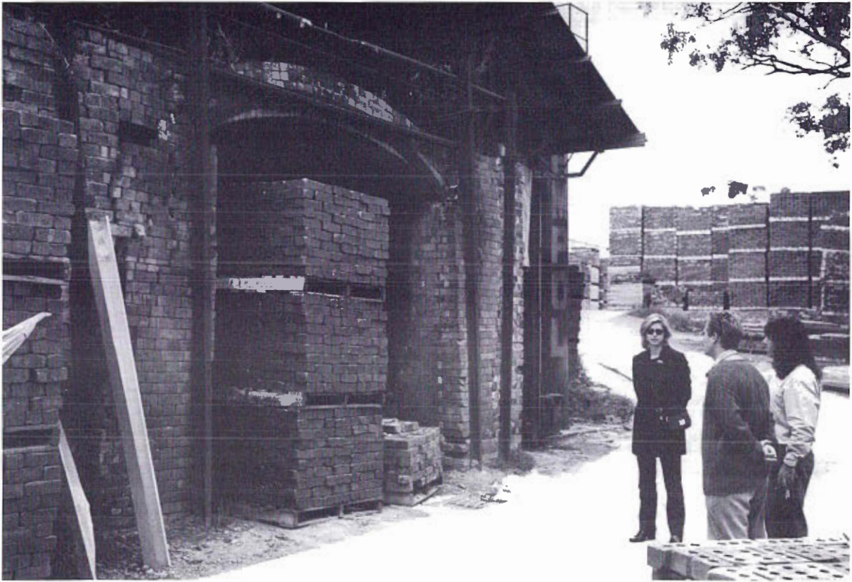
Littlehampton Brick Kilns in 1998. The kilns are now used as a storage area.
