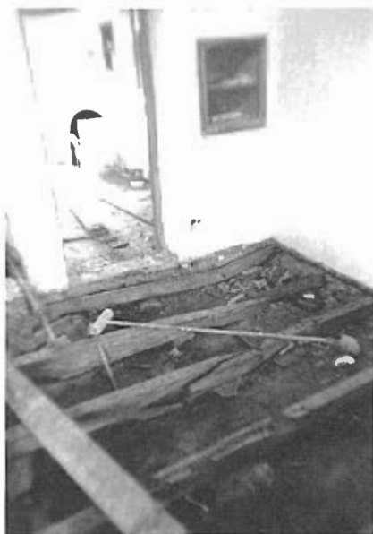
Left: Floor of stone cottage before reconstruction. Joists and dwarf walls were replaced and new footings added.
