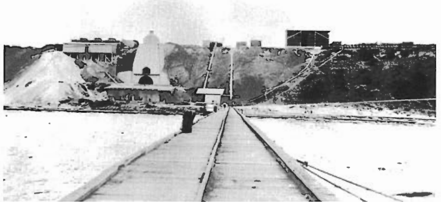
Above: Original lime kiln.
