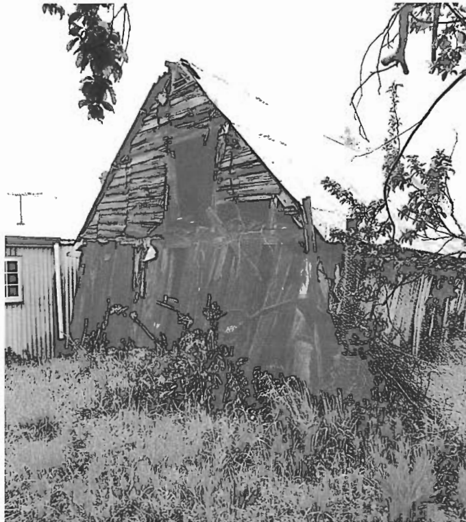
Left above and below: The Gare's timber cottage before and after.
