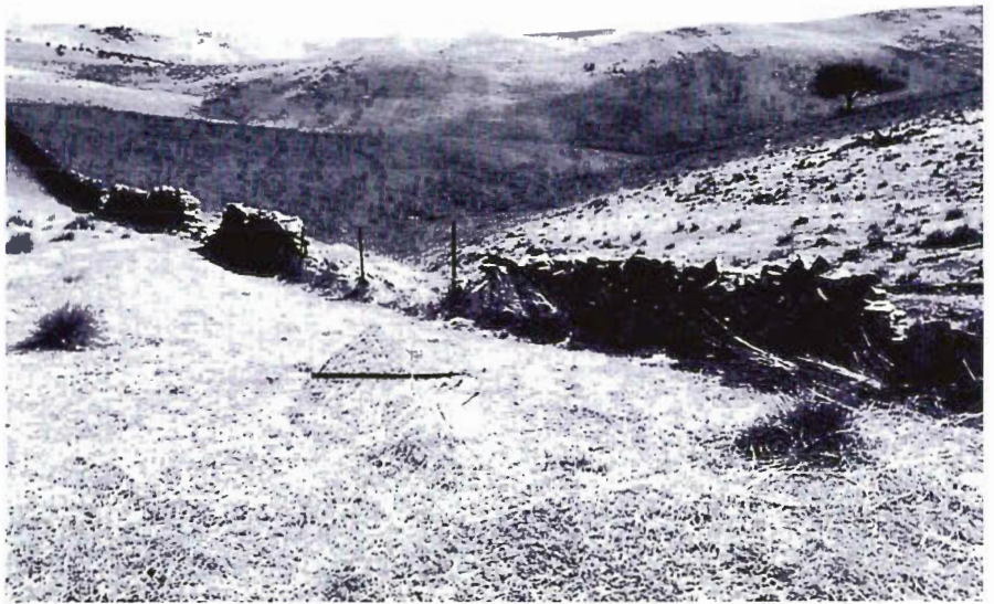
above: Wall in disrepair
