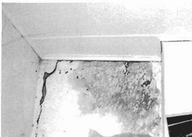
Left: An interior view of a corner depicting falling damp and cracking. These need to be repaired as a matter of priority.
