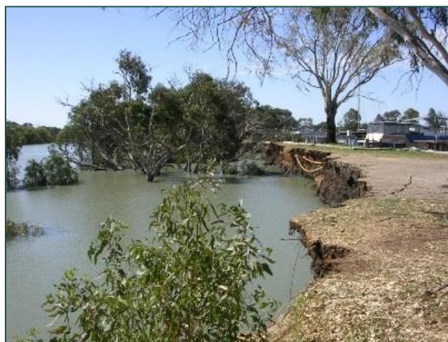
Riverbank Collapse – Long Island Marina 2009
