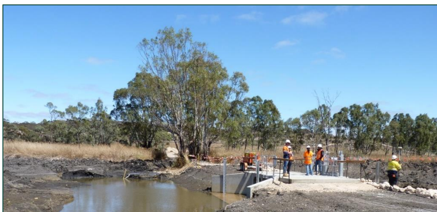
Construction of an environmental regulator
