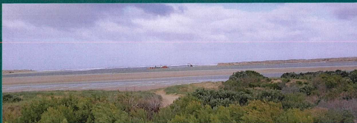
Dredging keeping the Murray Mouth open
