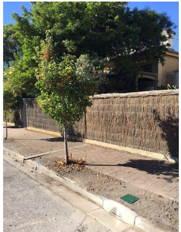
Figure 6. Tree inlet pits connected to associated underground soakage provides for passive use of urban runoff for urban greening
