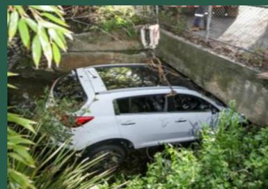
*Drains can also 'fail' for other reasons. This photo shows a car that has been swept into a drain, severely reducing its ability to carry away floodwaters. Other obstacles often encountered in drains include woody plants and other vegetative debris, and urban rubbish. Drainage management including removal of obstacles is an ongoing challenge, which can be further exacerbated where the responsibilities and powers for clearing drains is not well defined.*
