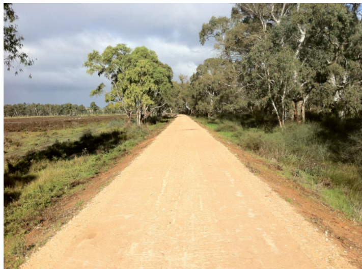
Cowirra Levee Bank
