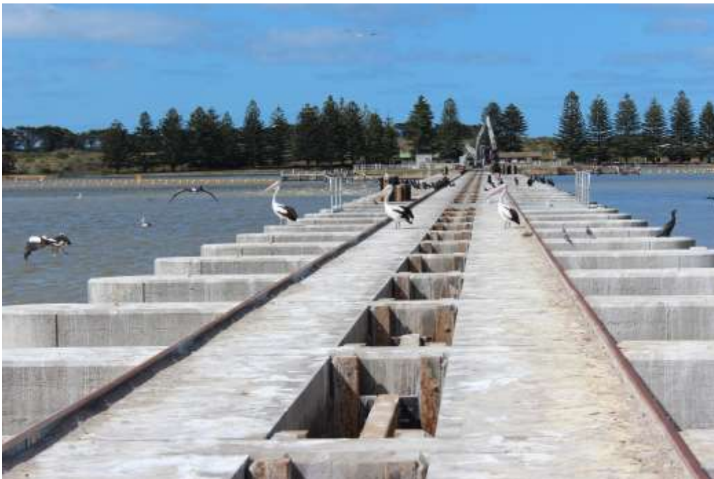
Goolwa barrage. Photo by Kirsty Wedge, DEW.
