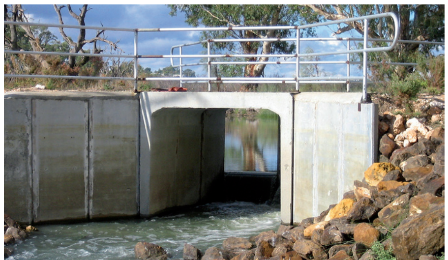
Outlet regulator at Schiller's Lagoon.
