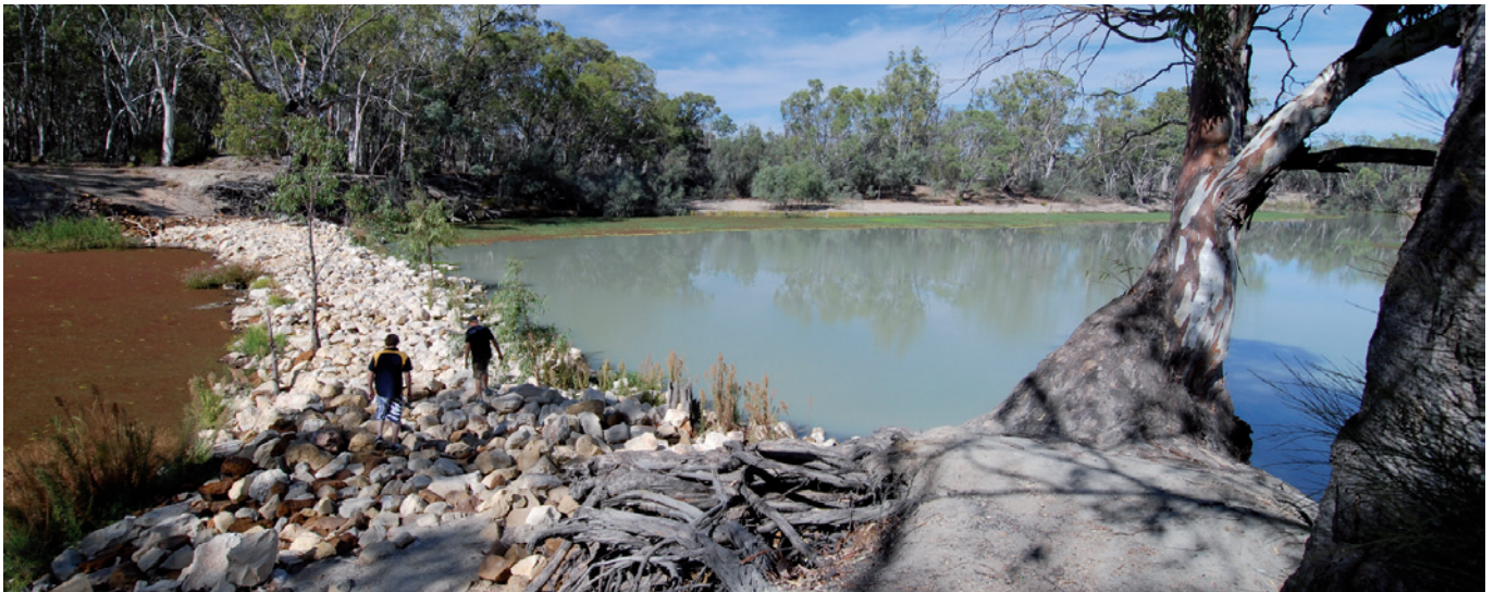
The Stone Weir is a major barrier to Katarapko Creek, and proposed to be modified to increase flow and fish passage.
