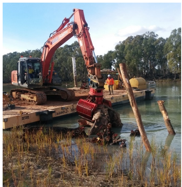
Figure 8: Moving of rootballs and timber to create new habitat in the main river channel
