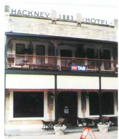
Painting of Older Buildings
