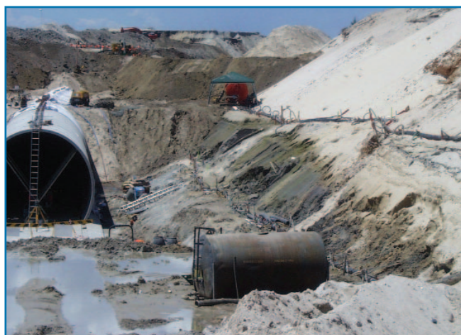
Figure 3b Exposure of buried potential acid sulfate soils at Barcoo Outlet, which were below the watertable and under sandhills.
