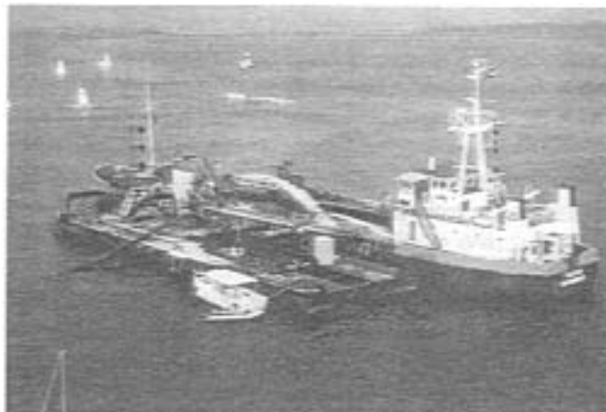
The Pelican Dredge used on the Adelaide Coastline
