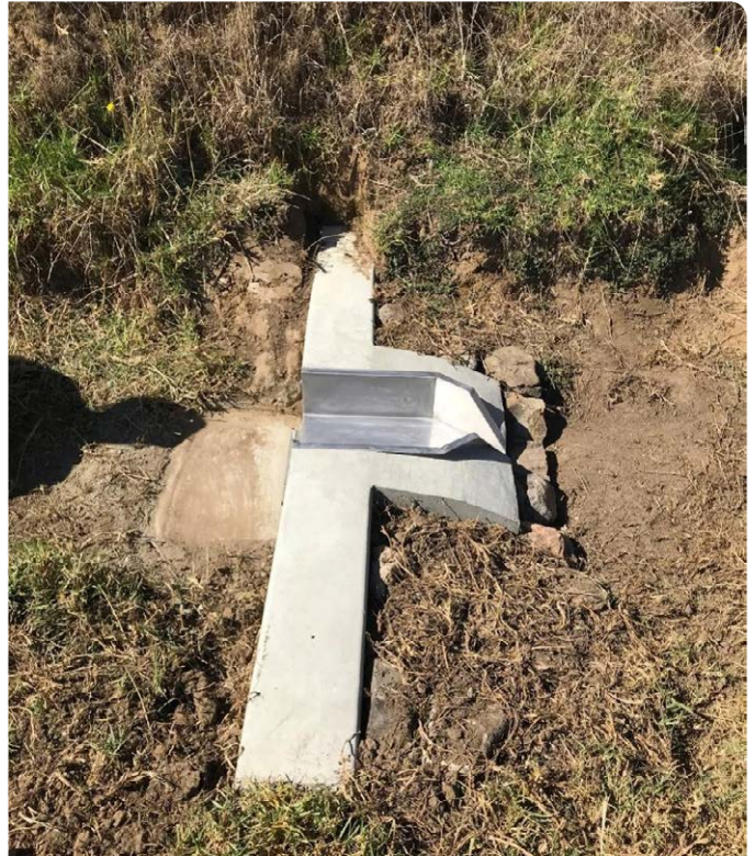
Release device inlet: A V notch weir is used to monitor inflows upstream of a dam.
