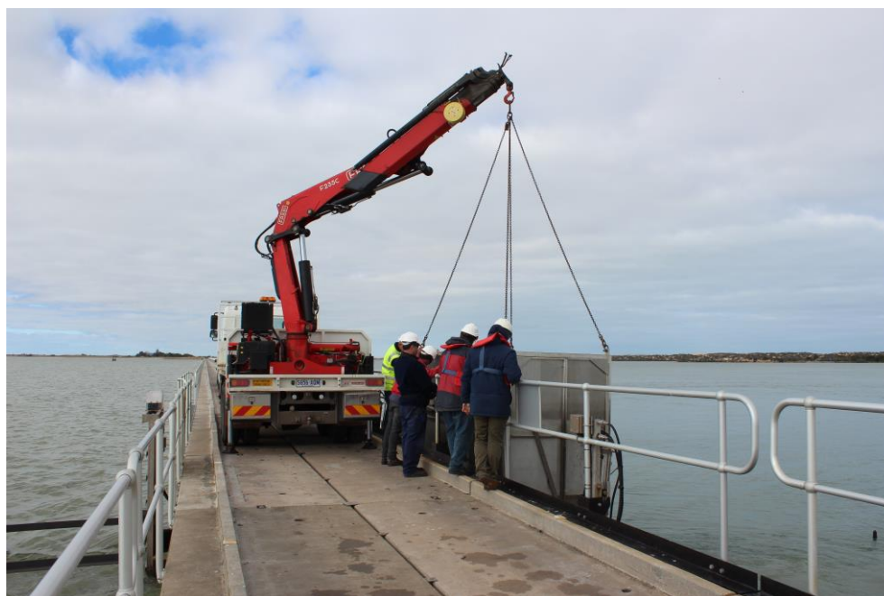
Figure 13. Crane pulling out a fish trap on the barrages, August 2016.
