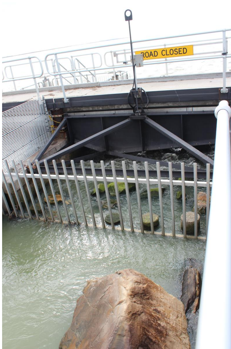
Figure 29. Tauwiche rock ramp.
