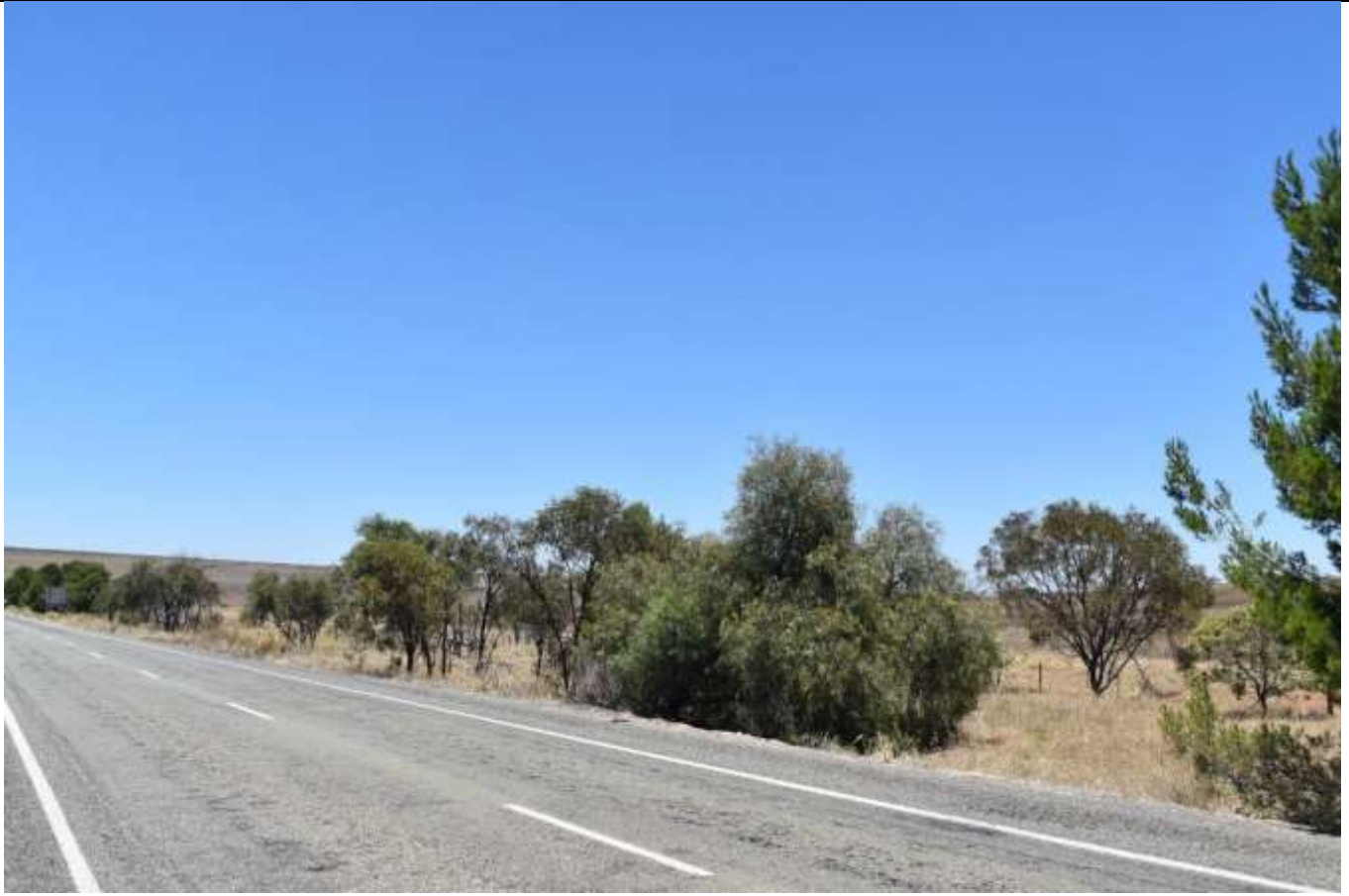
Photo 1. Looking southwest across the road reserve from approximate MM 151.0, RHS. GPS 264210/6269511. Impacted by hazard reduction and widening including fill batters.
