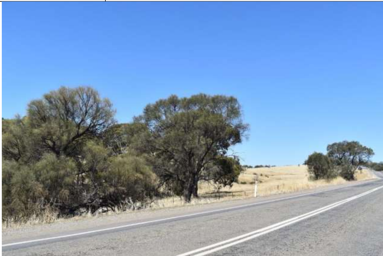
Photo 3. Looking northeast from approximate MM 159.5 GPS 271712/6267237, LHS. Impact is due to hazard reduction (proximity to road) and/or drainage upgrade.
