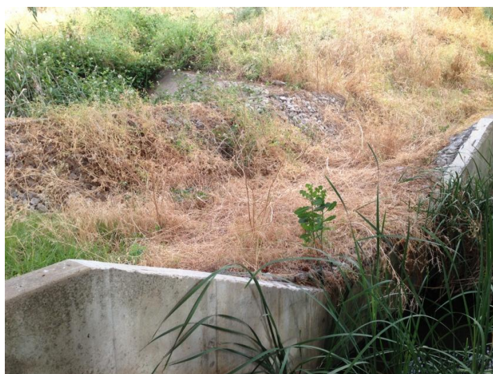
Figure 10 Former Aqueduct Channel passing over watercourse (Catchment 12)
