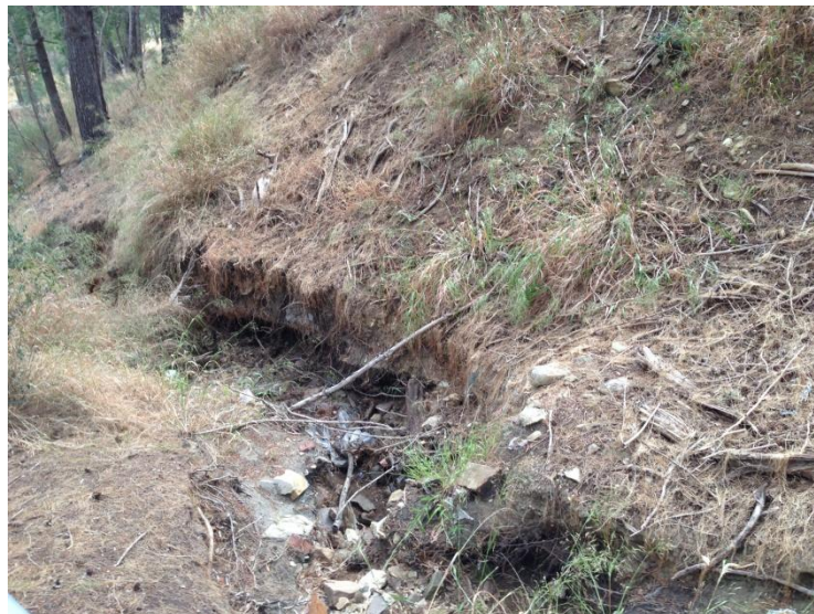
Figure 8 Deeply eroded gully (Catchment 9)
