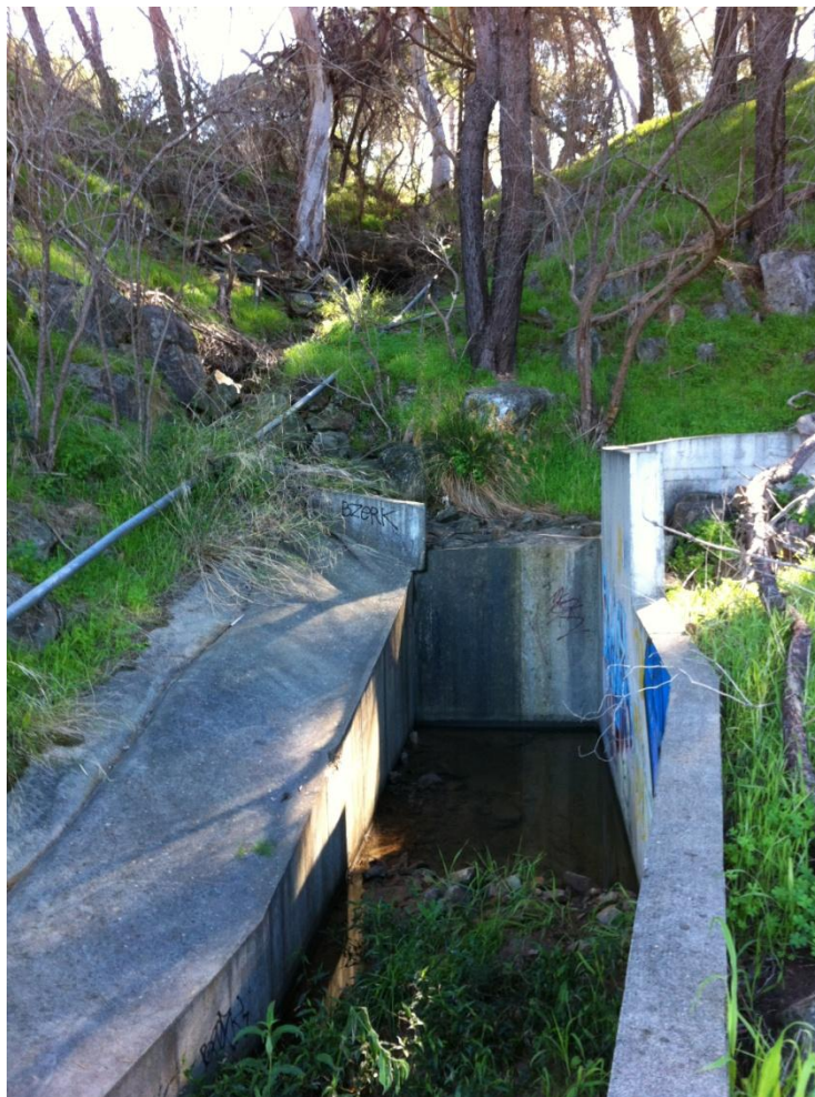
Figure 7 Existing concrete drop structure (Catchment 5)
