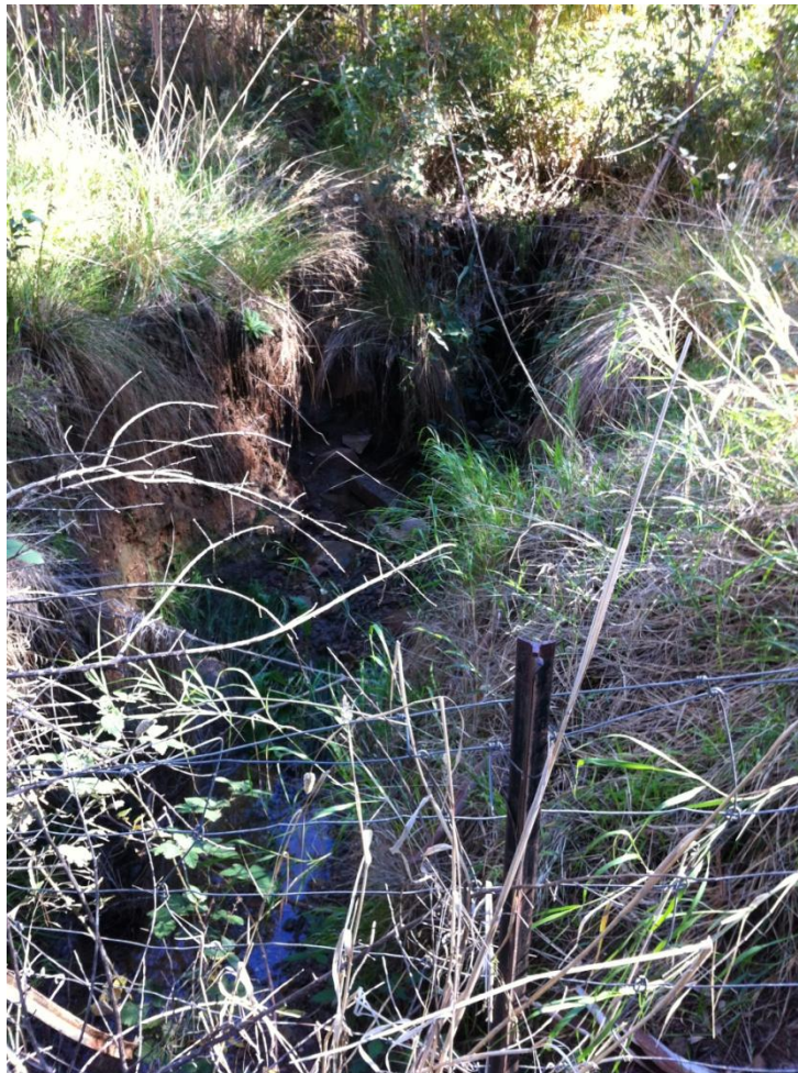
Figure 5: Channel Erosion, immediately upstream of the southern cliff face (Catchment 5)
