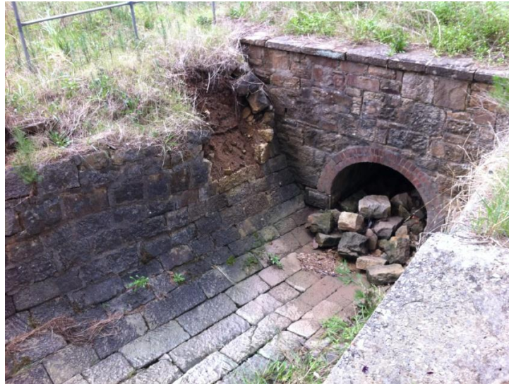
Figure 9 Original Aqueduct Underdrain Structure (Catchment 10)
