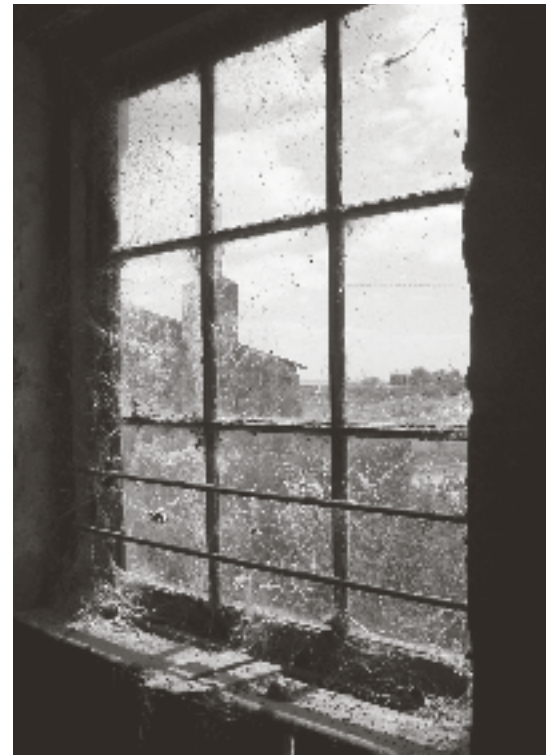
Poltalloch Station Shearing Shed window
