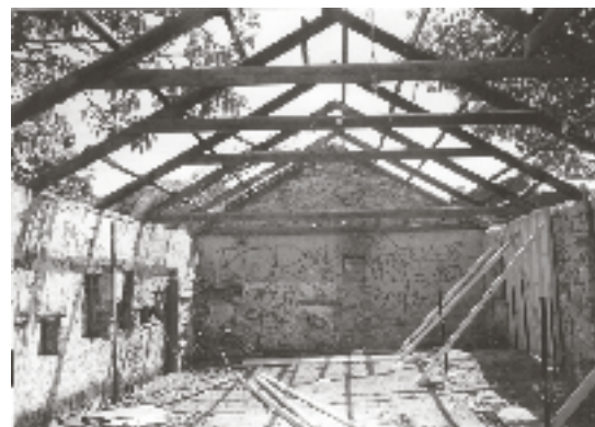
Former Reynella Changing Station Stables, before restoration work
