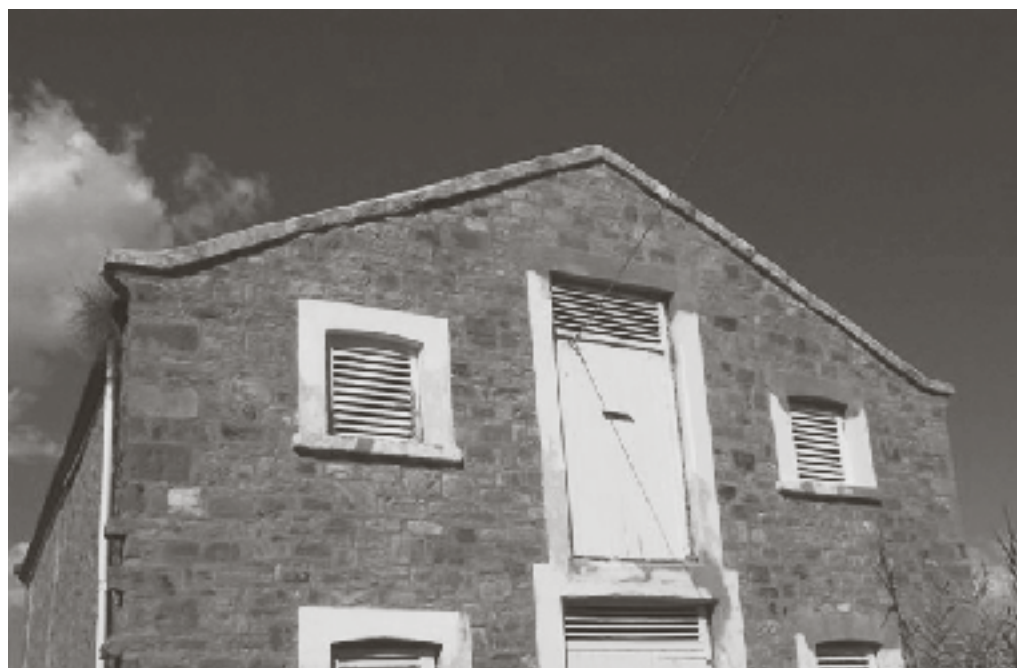
Former Coaching Stables, Wilmington, after conservation work
