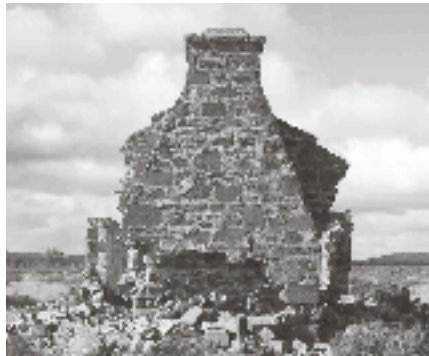
Pondana ruins before stabilisation work
