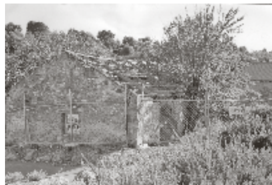
Former Reynella Changing Station Stables, before restoration work
