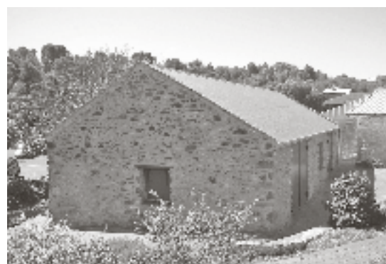
Former Reynella Changing Station Stables, after restoration work (photograph by Malcom Harrington)
