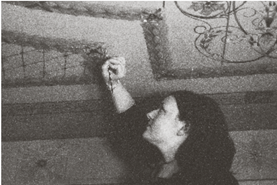
Conserving the ceiling of the Summer Sitting Room, Ayers House
