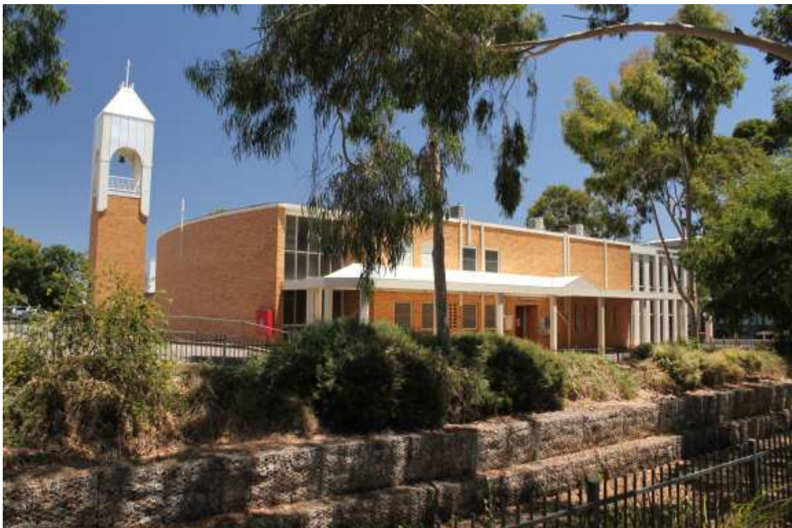
View from northeast showing tower; note post-1999 tower belfry. Source DEW files 2021.
