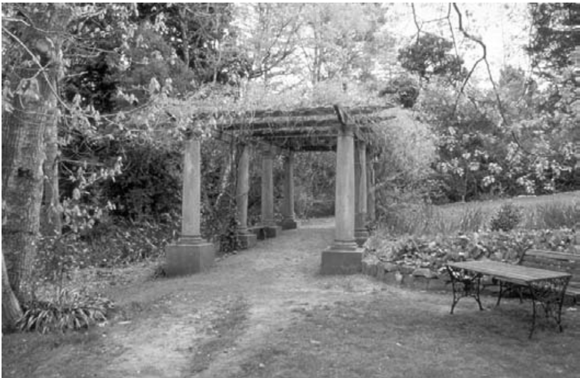
Wisteria covered concrete and timber pergola at 'Drapers Hill' Crafers. Source: David Jones 1997.
