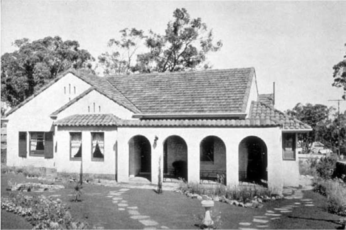
A Spanish Mission style house: Mr & Mrs AN Bartrop's residence in Portrush Road, Glen Osmond. Source: South Australian Homes & Gardens, February 1, 1938, p. 38.
