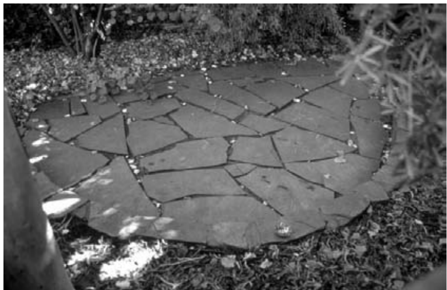
Mintaro slate crazy paving constructed by Robin Hill in 1964 in Frewville. Source: David Jones, 1997.
