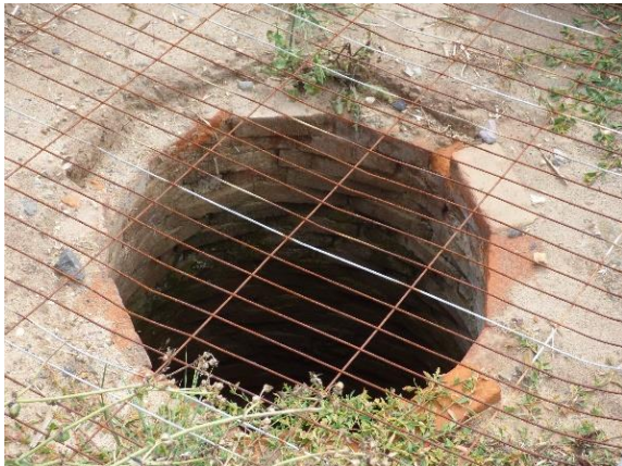
Uncovered well 23 November 2017 Source DEW
