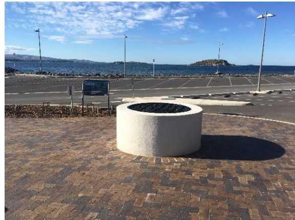
Site works complete June 2019 Source DEW
