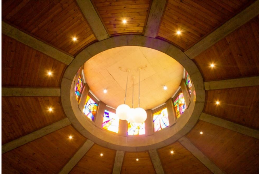
Inside of roof lantern showing coloured glass and replacement light fittings
