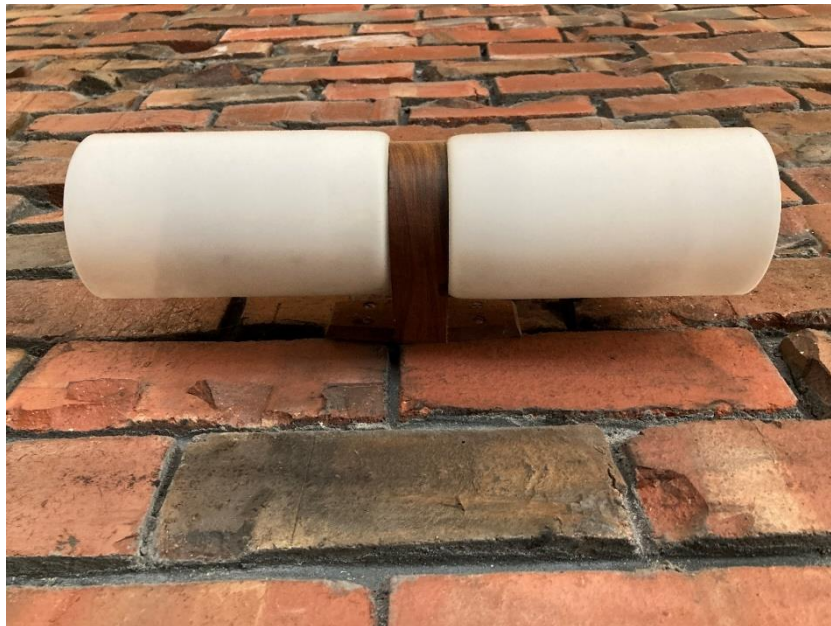
Original light fitting in chapel
