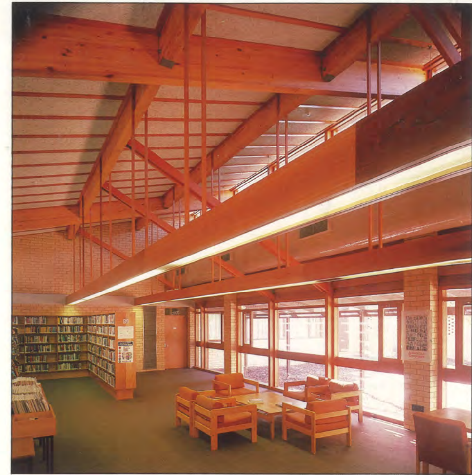
Interior, looking out to forecourt. Strip lighting is housed in western red cedar channels.
