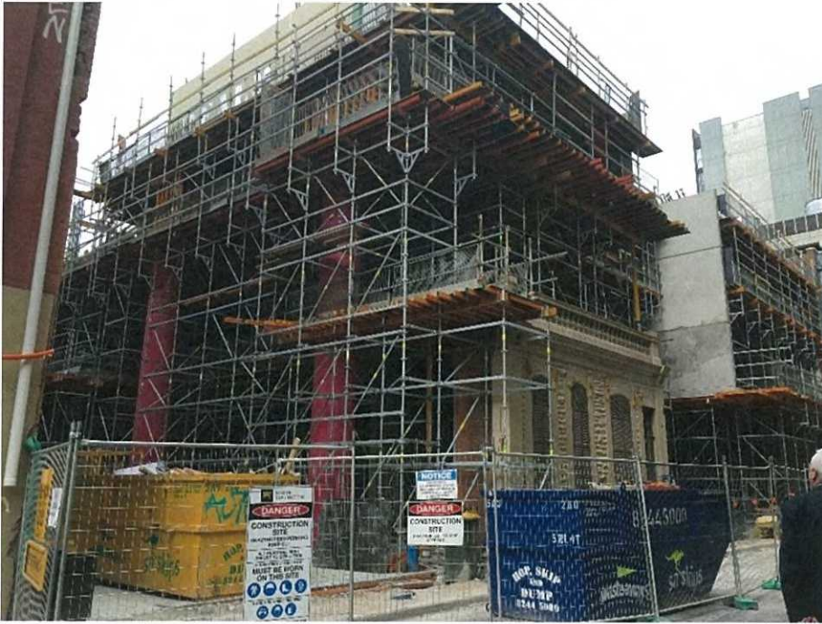
Figure 7. The former Assay House, Austin Street, Adelaide. The façade of Assay House, a local heritage listed building, has been retained, but the rest of the building has been demolished for high density accommodation.
