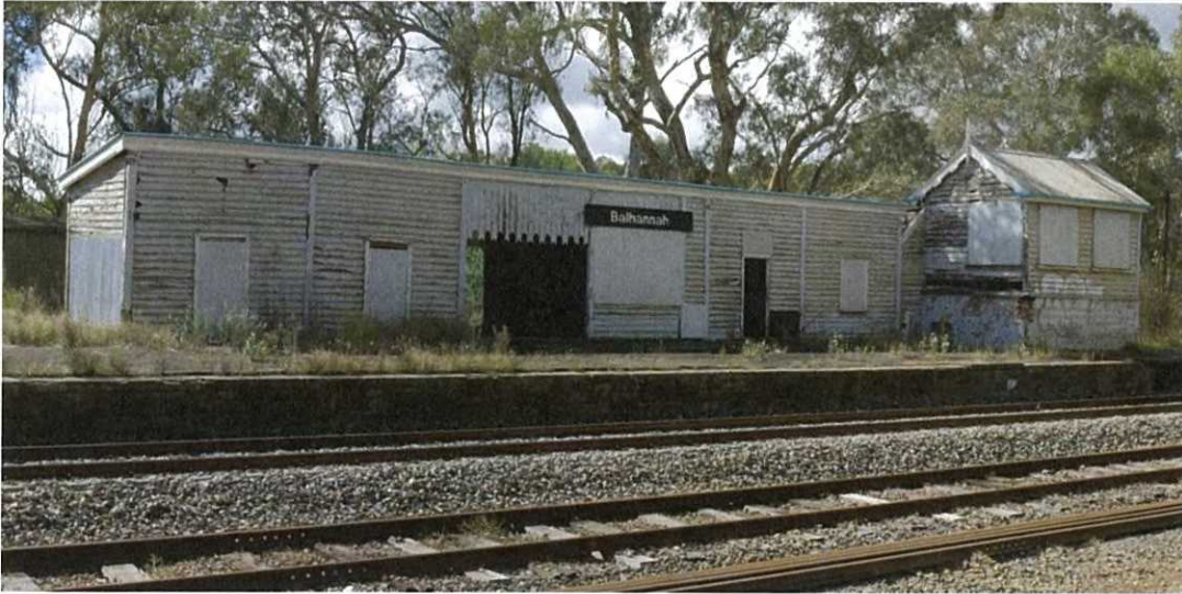
Figure 9. Balhannah Railway Station and Signal Cabin (SHP 12854) – an opportunity for heritage building conservation training? (SA Heritage, Department for Environment and Water, 2018, p. 2)
