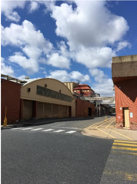
View of brewery buildings with the Brewhouse Tower.
