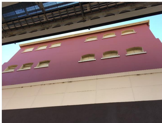
Southern elevation (facing Winwood Street now closed)
