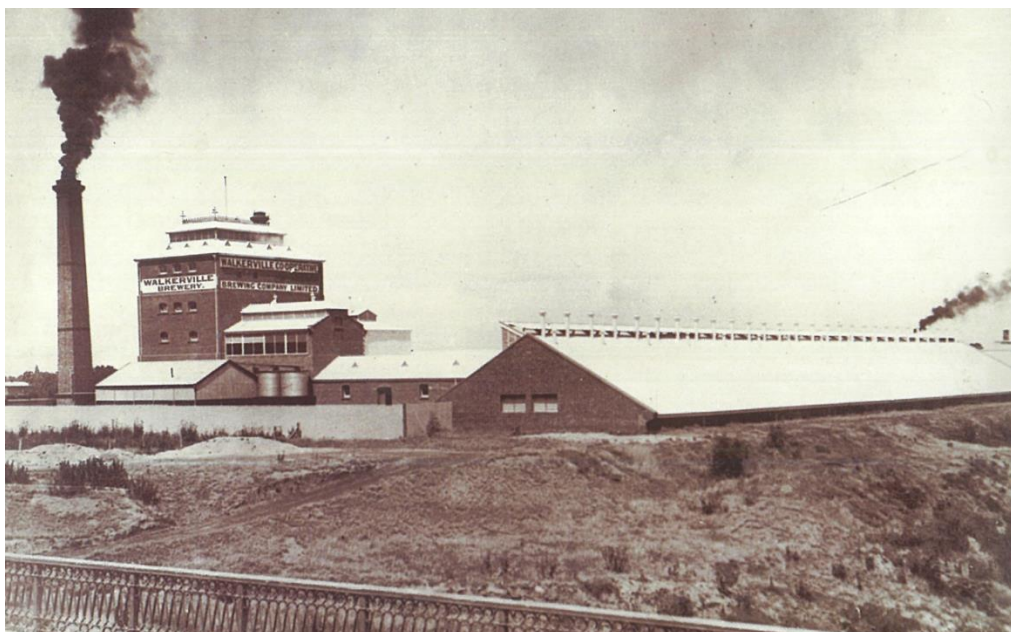
Walkerville Brewery c.1903 showing the doubling of the brewhouse and tower and new facilities at the brewery (to the east of the site). The chimney bellowing smoke is a new addition (the original can be seen just peaking over the top of the tower roof).
